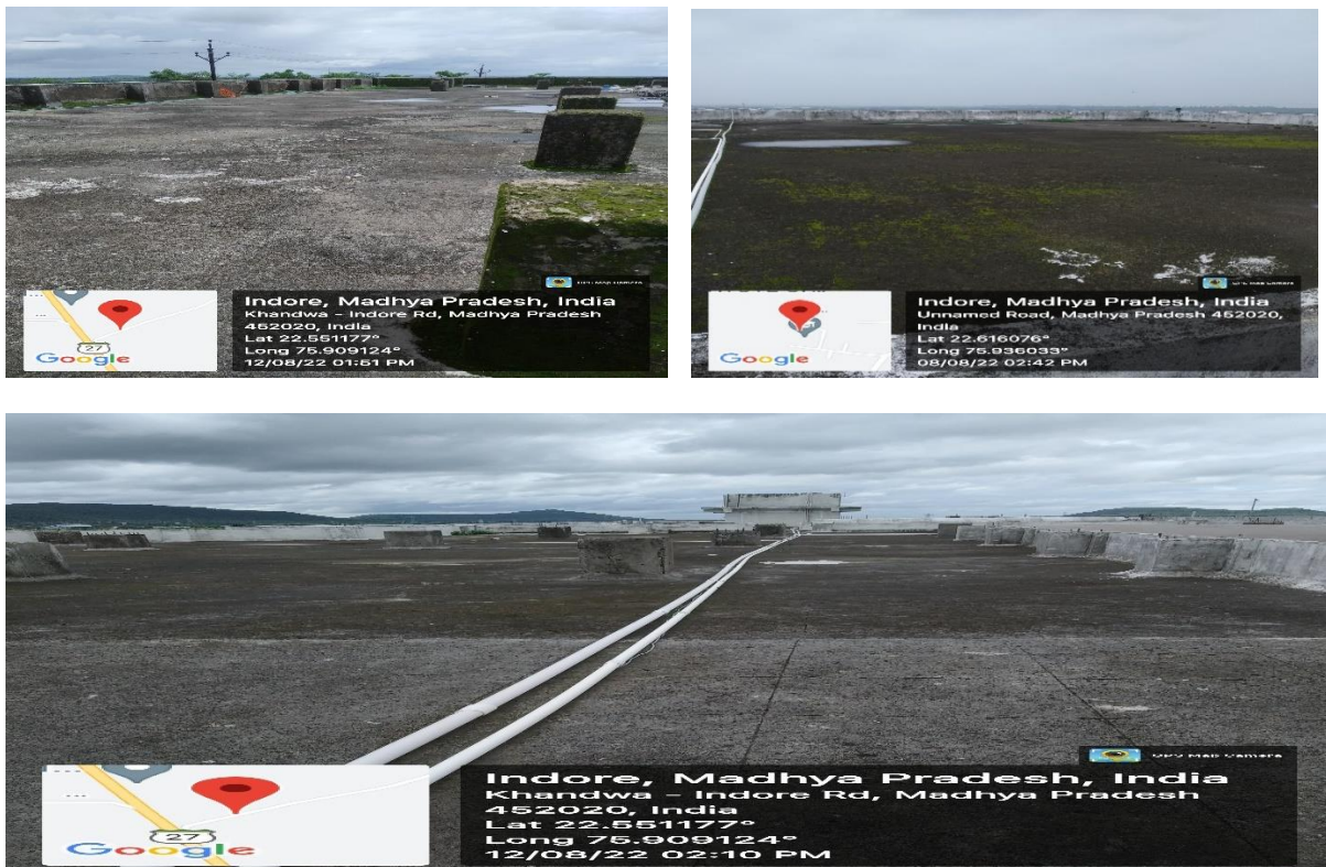
Fig.: 3.2 Roof top of institute buildings
